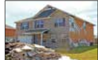
Note that roof covering damage is not visible in the photograph. The resulting interior water damage is indicated by the yellow stain near the roof.
